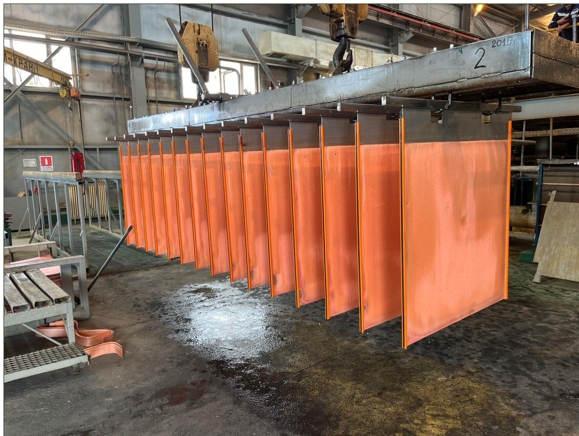
Figure 16-9: Copper Cathode Harvesting
