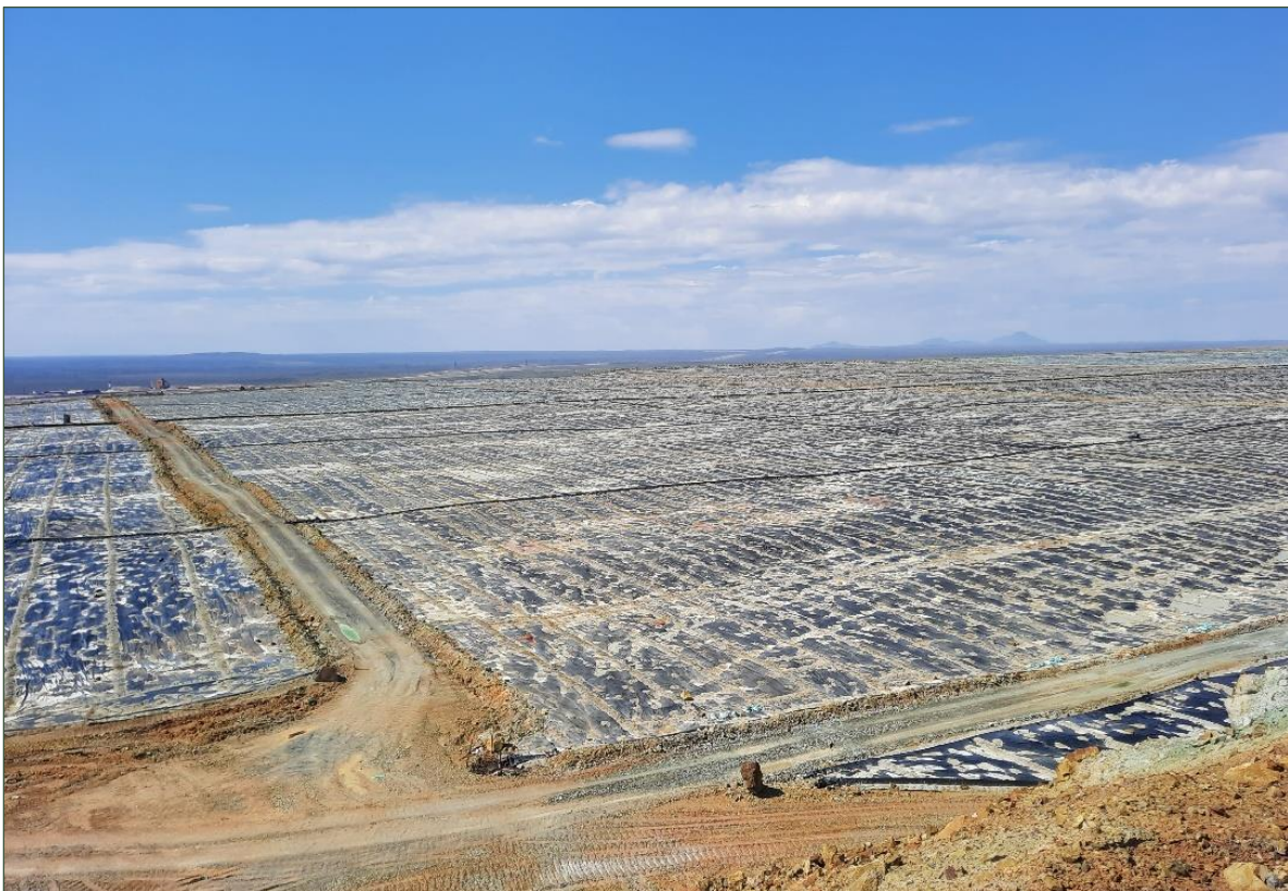
Figure 16-3: Winter Leach Pads using HDPE Liner
