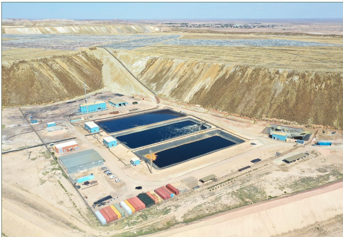
Figure 16-5: Western Dumps Collection Ponds, Boiler Houses and Pump Stations
