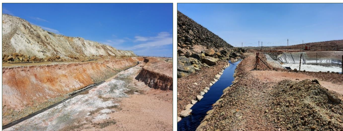
Figure 16-4: Leach Solution Collection System
