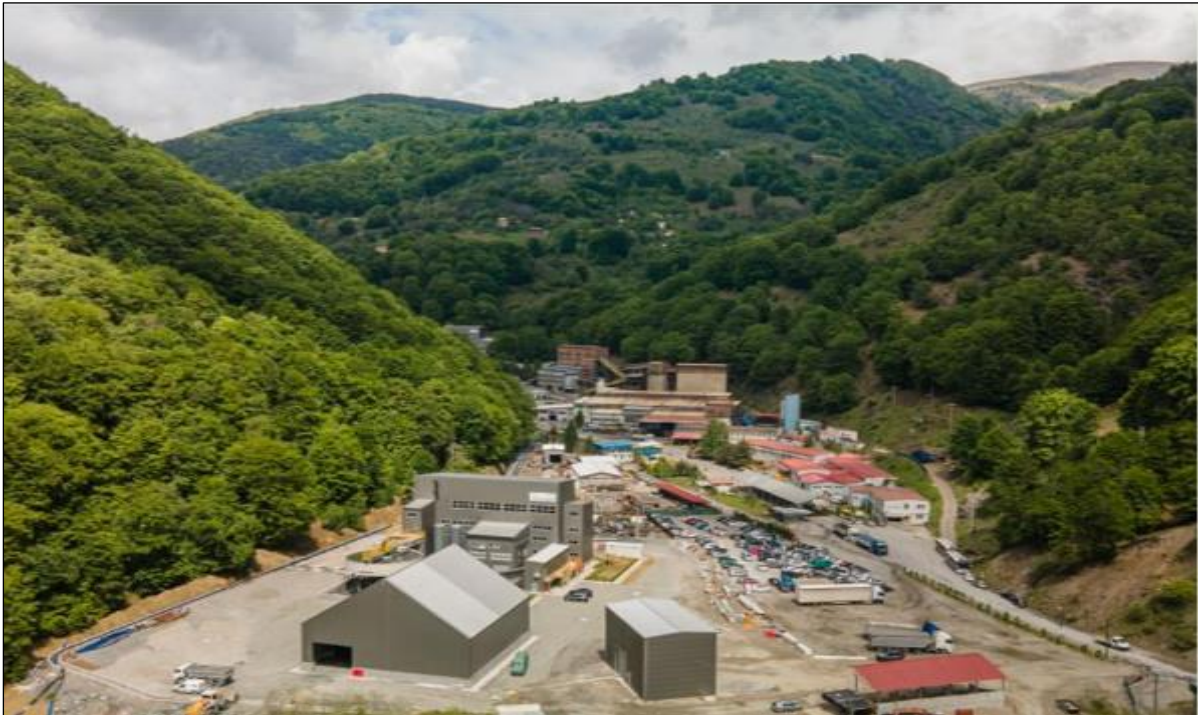
Figure 4-3: View Looking Northwest of Sasa Mine Surface Infrastructure
